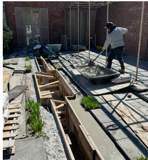
Flowing Through Time: Restoring the Inner Garden’s Historic Rill The Inner Garden Rill is once again an aesthetic delight. Wethersfield had to remove and re-pour its concrete foundation and repair its broken irrigation system. It is now beautifully replanted, with the lovely sound of gently moving water.
