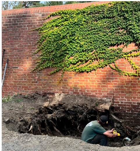
The western wall of the Inner Garden This wall has been re-braced with buttresses for stability and visitor safety, after tree roots had undermined its foundation. This area is now reopened to the public, and is graced with overhead grapevines for shaded seating, punctuated with hanging baskets of bright fuchsia.
